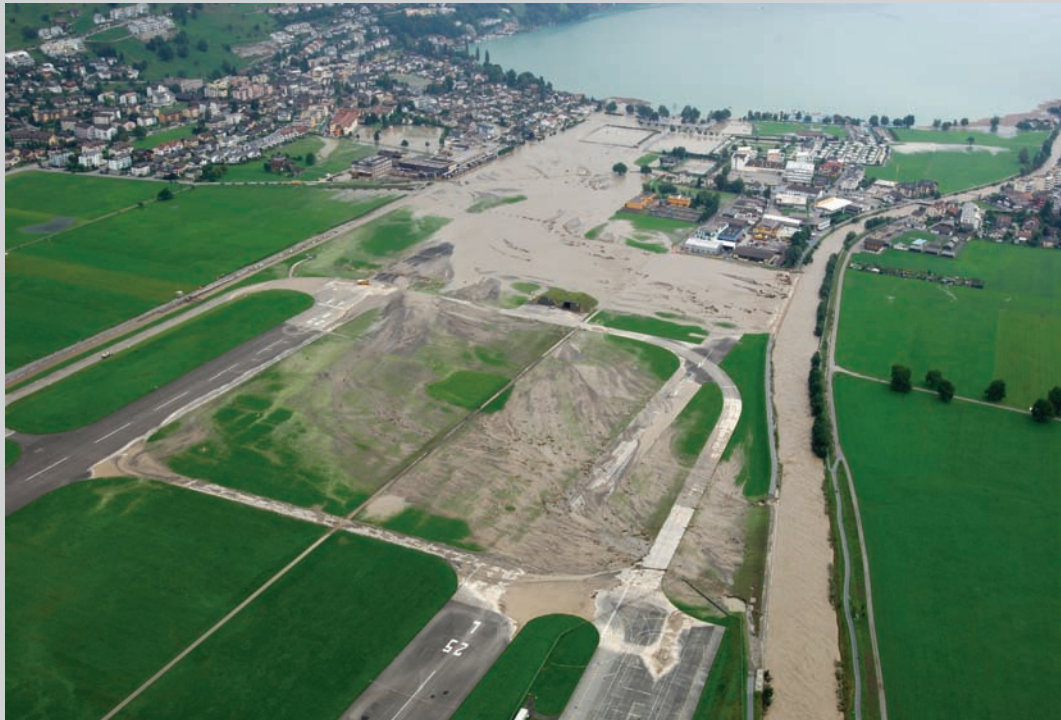
Figure 3: In August 2005, the flood of the Engelberger Aa was redirected around the vulnerable settlement area. (Source: Swiss Air Force 2005)
